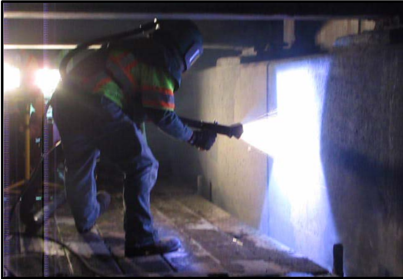
Spraying Al-Zinc Anode Coating to Surface
